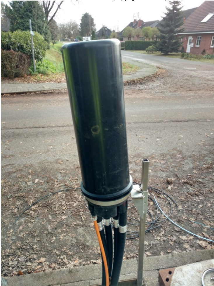
Photo 2: Pressure-sealed splice closure (copyright: ElbKom)
