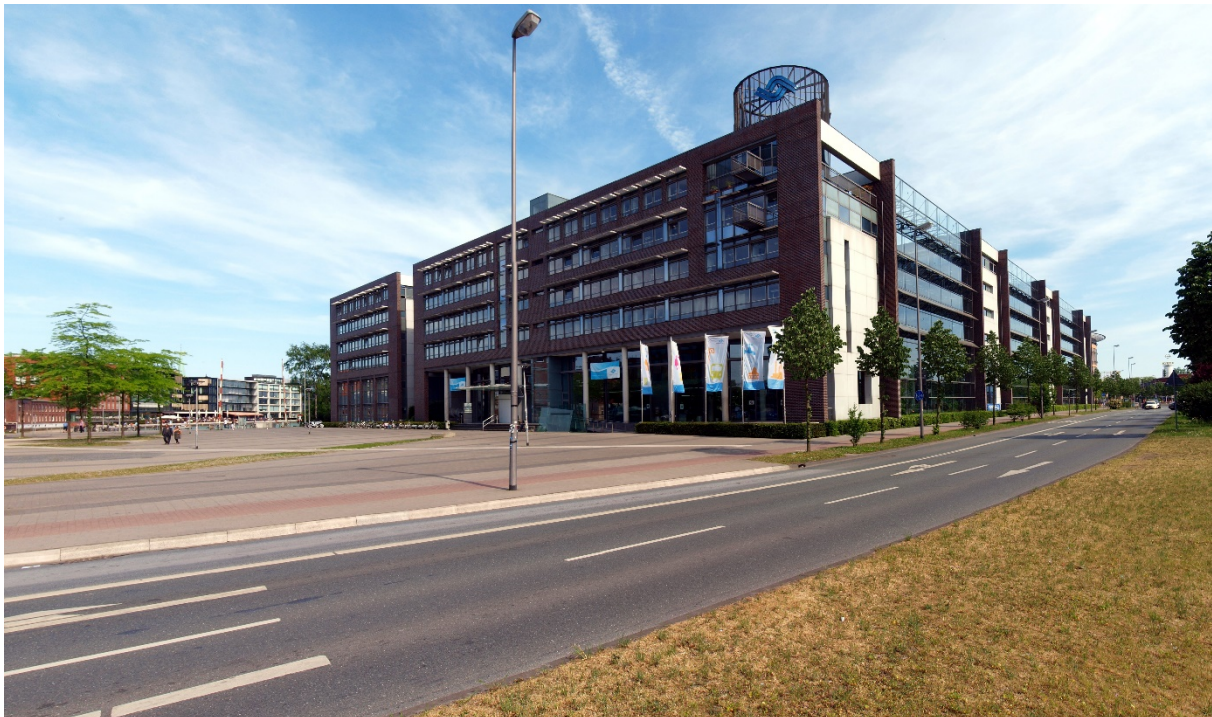
Photo 1: Main building of the utility Stadtwerke Münster (© Stadtwerke Münster)
